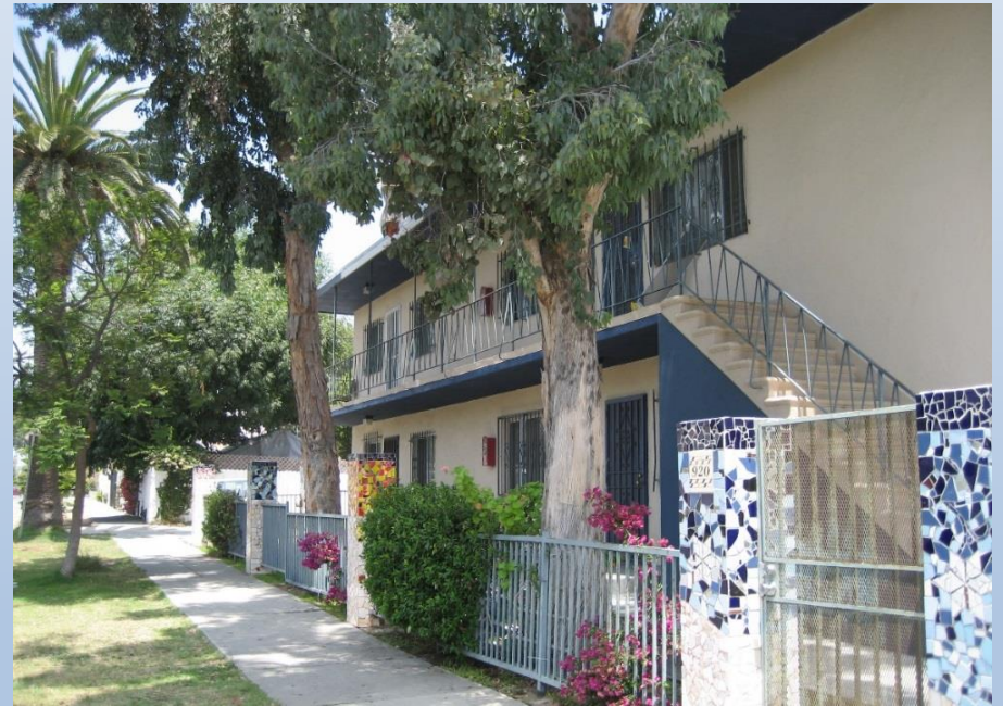
Rehabilitation/Preservation, Affordable Housing 6 th Ave, Venice
